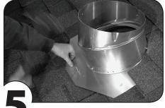
Slide top half of flashing under entire perimeter of hole with roofing cement. shingles. Secure with nails at top, sides and by turning counter clockwise. bottom.
