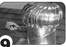
Position the Whirlybird® turbine holes in the brackets and elbow and fasten with sheet metal screws.
