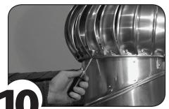
After installing, check to see that Whirlybird® turbine vent turns freely. In transportation it may have shifted slightly. If necessary, minor adjustment may be made by gently prying lowest point of turbine upward to remove any wobble.
