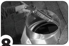
$\bullet$ Seal the adjusting seam and the base/elbow connection seam on inside with head on the base. Line up the predrilled roofing cement. Seal locking clamp holes and all exposed nails with roofing cement.
